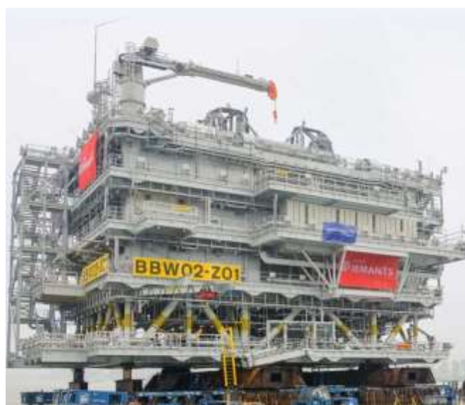
Figure 5.2: Burbo Bank Jacket and Foundation
